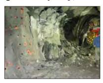
stone, concrete and reinforced concrete. "Dā-mite is mixed with water and placed in the appropriately placed predrilled holes, where it sets and expands, fracturing the rock/concrete". No license required. There are four grades of Dā-mite, providing enough versatility to be utilized in drilled hole diameters from 1 in. to 2 ¾ in.
