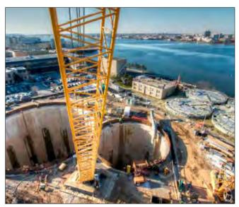
DC Clean Rivers Project, Washington, DC: Division A - Blue Plains Tunnel, reinforced concrete slurry diaphragm wall shafts (pictured); and Division I Diversion Structure, jet grouting for underpinning, support of excavation, and groundwater control
